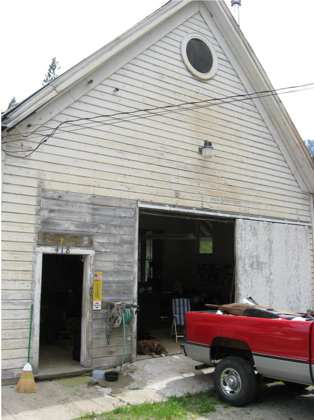
North façade prior to rehabilitation work after 2009 (Photo: Nora Prince collection)
