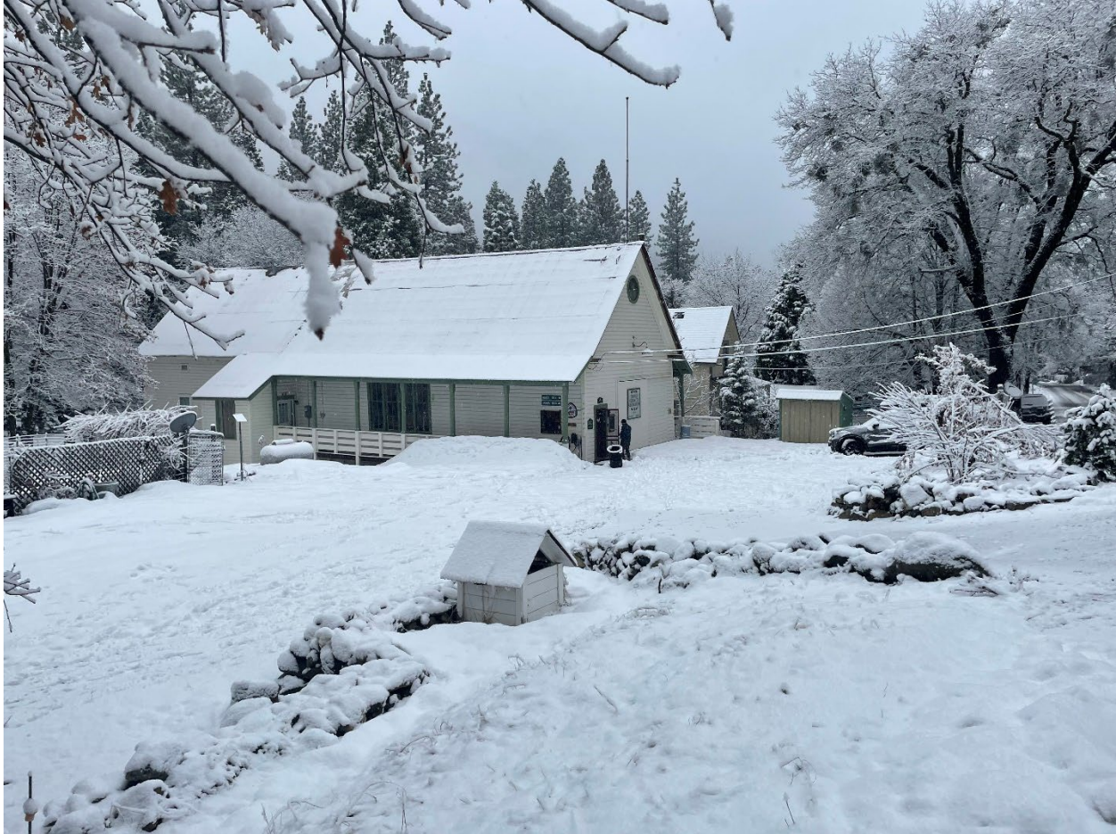
Photo 0002 - Looking at NE corner of Sierra City School or Highway 49 (Main Street)
